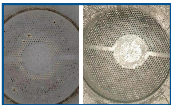
Figure 1 : Before and after cleaning pictures tube side
